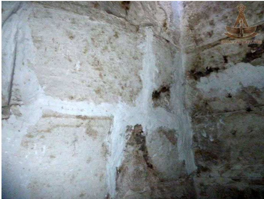
Views of plaster repairs
