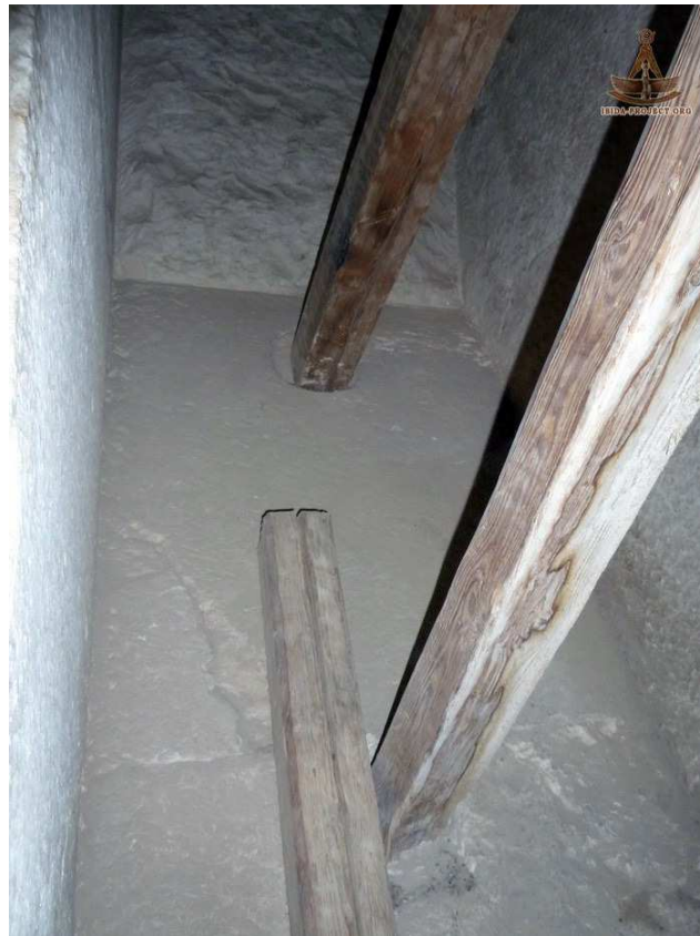
Eastern portcullis supported by modern beams.
