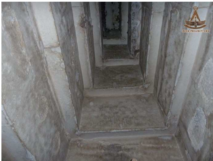
Close up view of the upper corbels.
