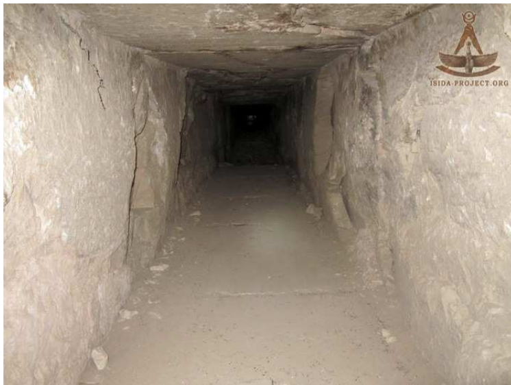
View up western corridor from the pit.
