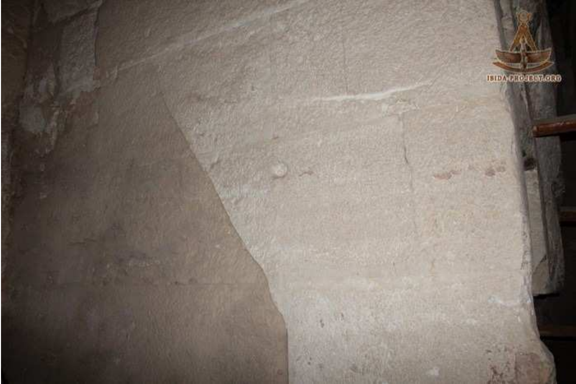
View along north wall, entrance is to the right.
