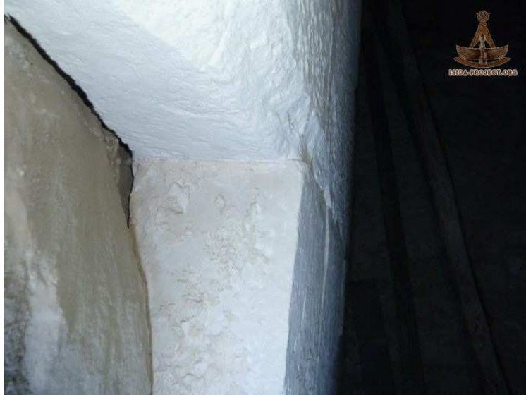
Closer view of what appears to be thick tiling.
