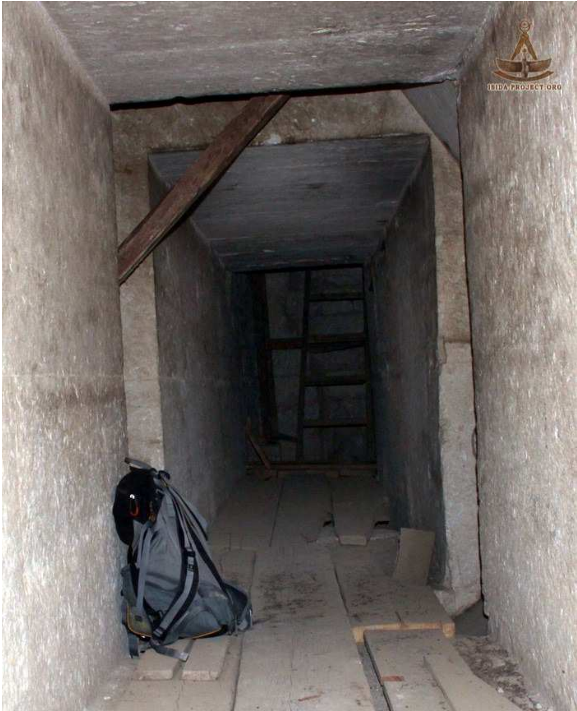
View looking east, with portcullis in stored position; the ladder in the background, leads to the top of the masonry massif, that was built inside the upper chamber.
