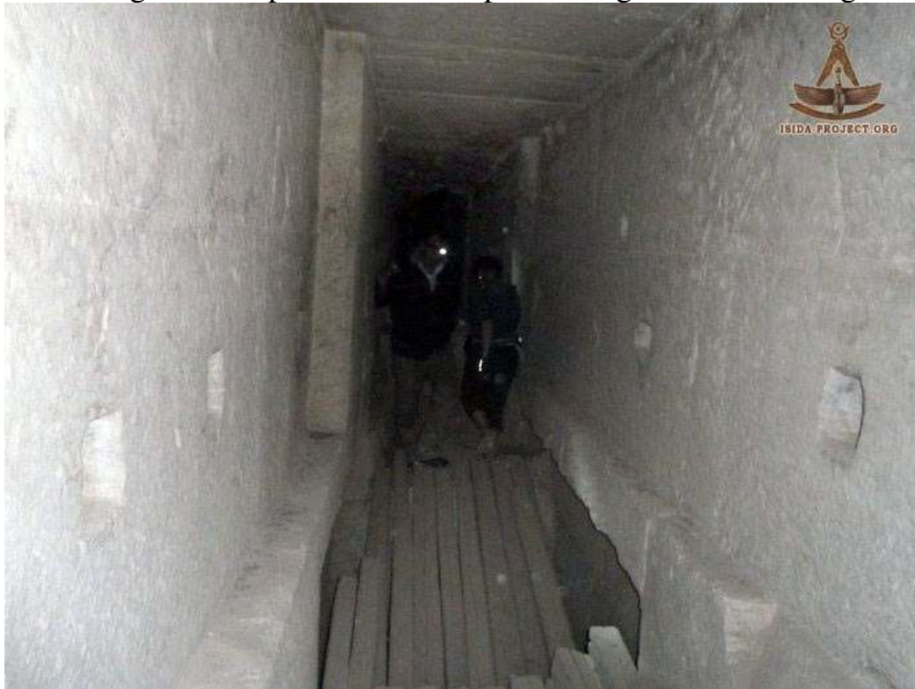
View looking east, wooden planks cover shaft.
