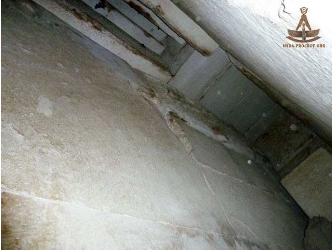
Views looking up into the western portcullis housing, the square block in Perring's drawing is visible to the right.
