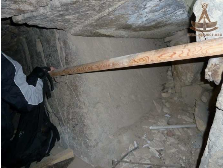
A view into the excavated west wall, showing the face of the continuous joint; also in view is the dressing of the roof mentioned by Petrie.
