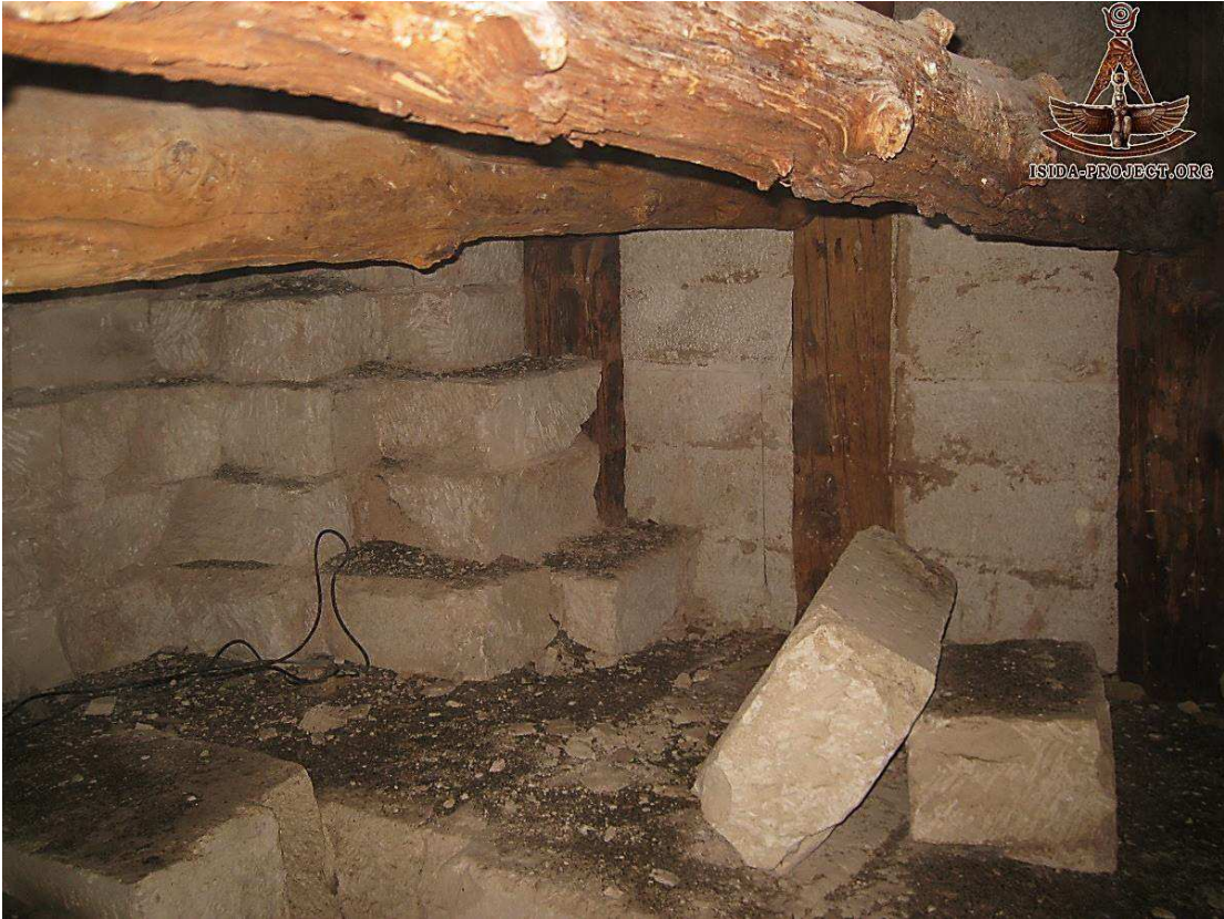
Blocks resting on chamber floor and good condition corbels
