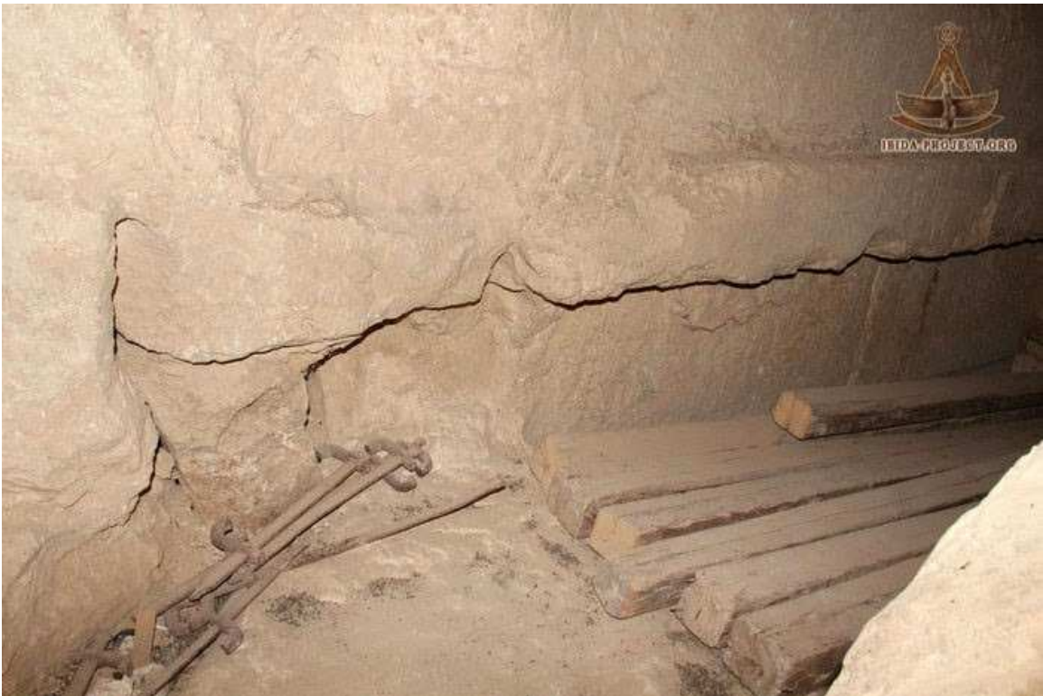
View from tunnel entrance with shaft to the right.
