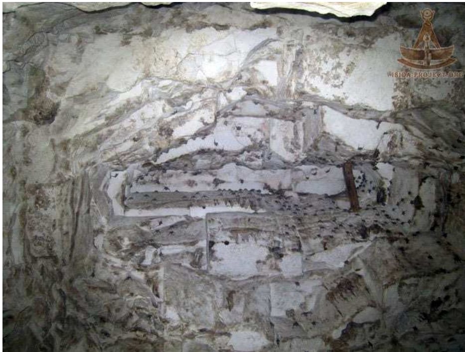
A faint glimpse of surviving corbelling exists at the top
