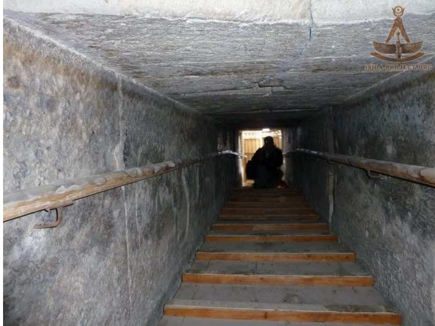
Looking up the north passage, Puchkov states the walls are made of a single course from the continuous joint.
