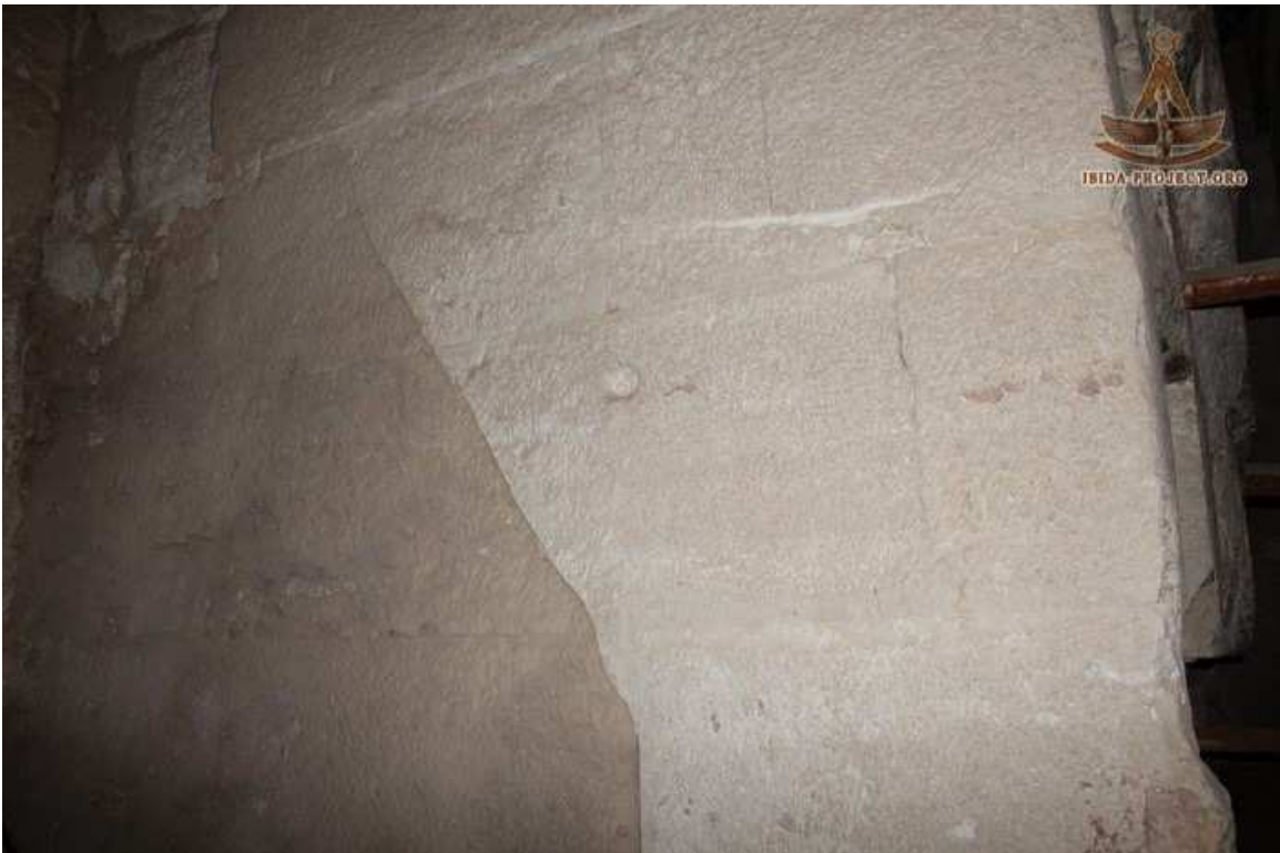
View along the north wall.
