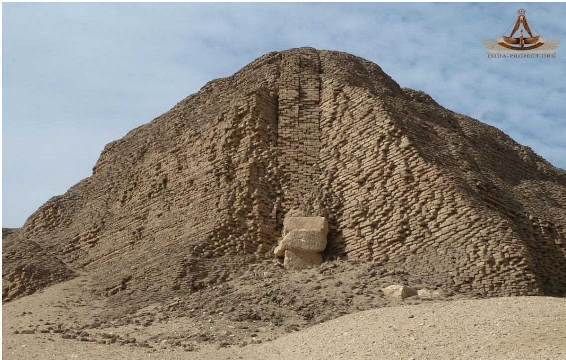
Two examples of diagonal brick walls laid on stone walls
