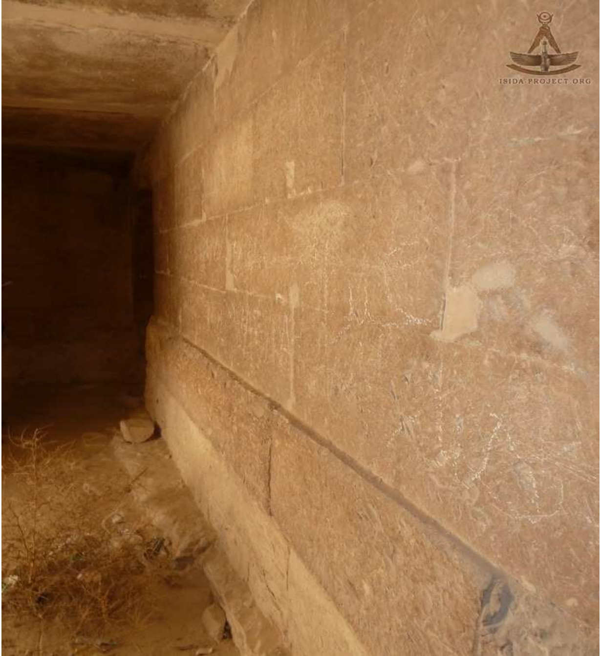
View along chamber east wall
