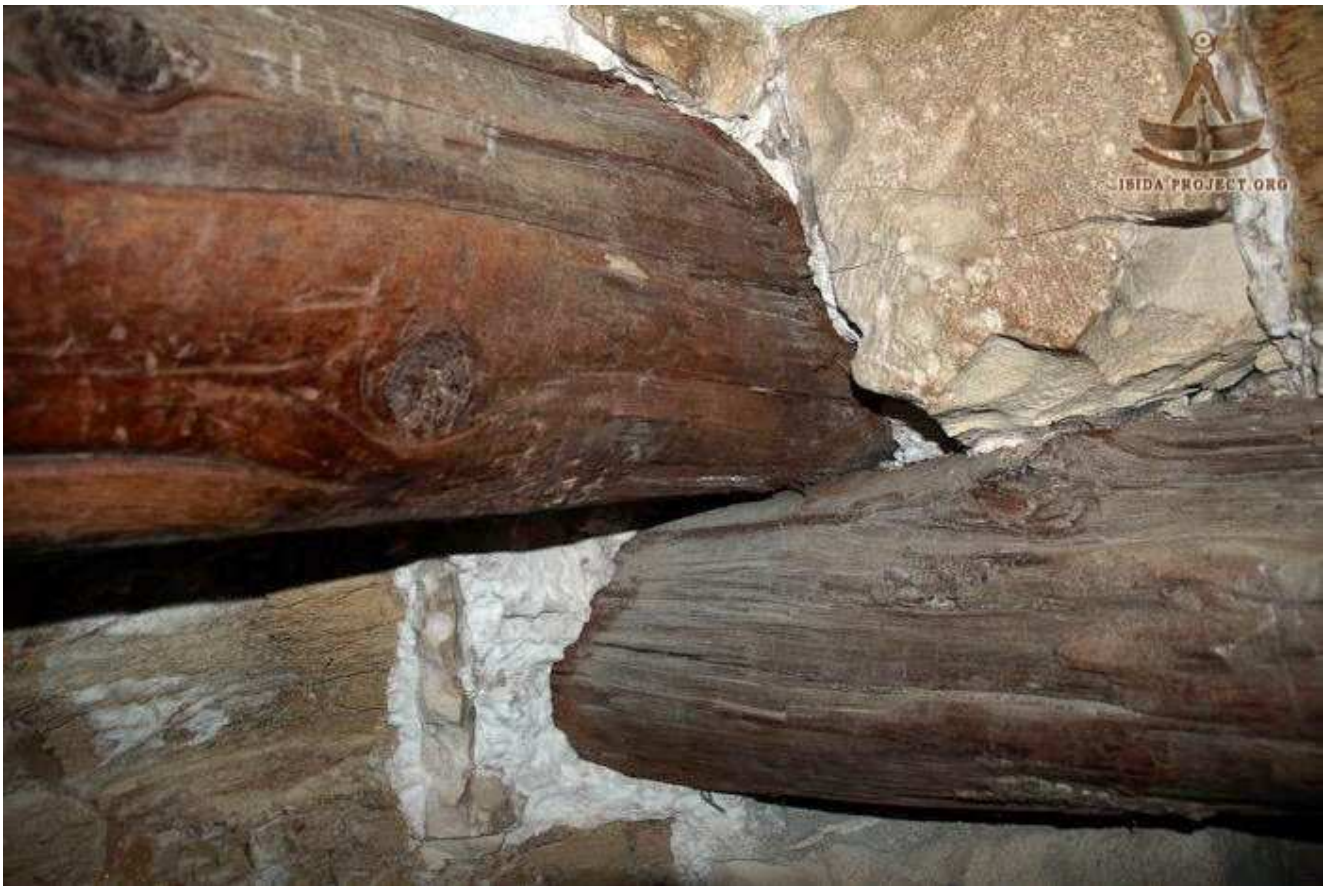
A close up view, where West and South wall beams meet
