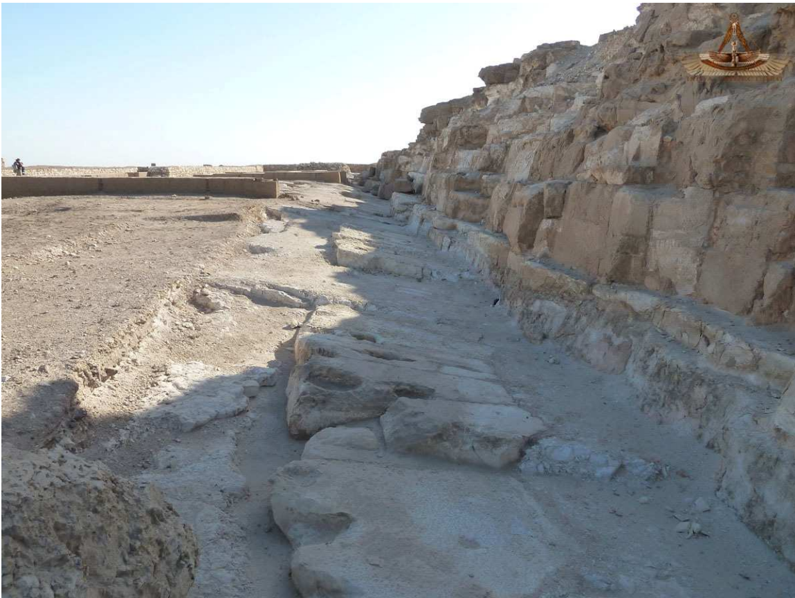
Sloping foundations east side, with possible notches/cavities
