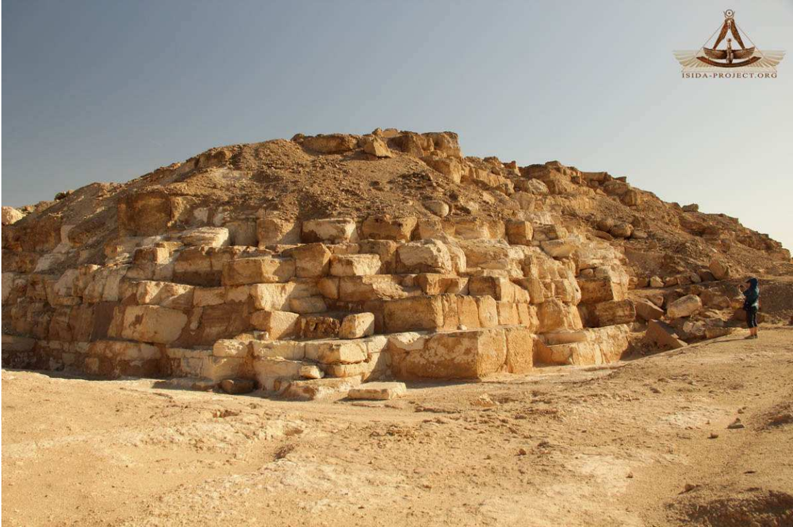
View of masonry, N.E. corner
