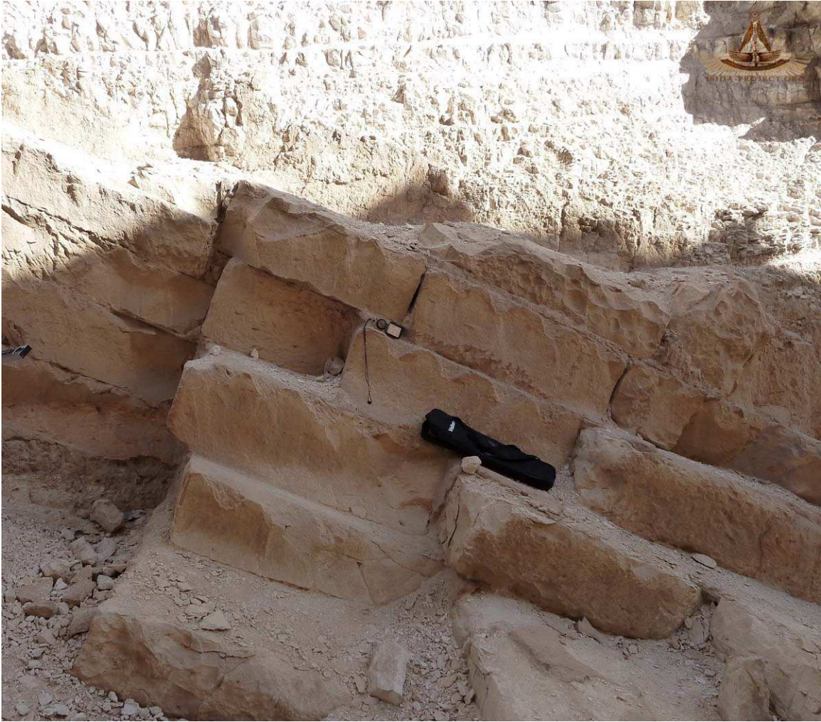
Section of trench floor and five courses of fine limestone
