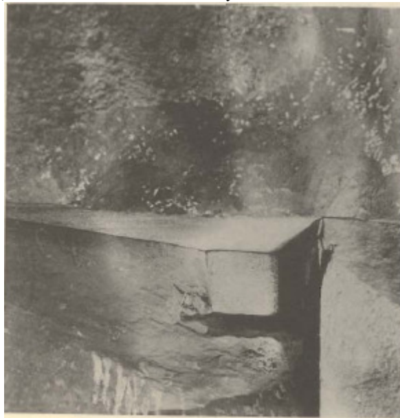
Close-up of dovetails position in north-east corner
