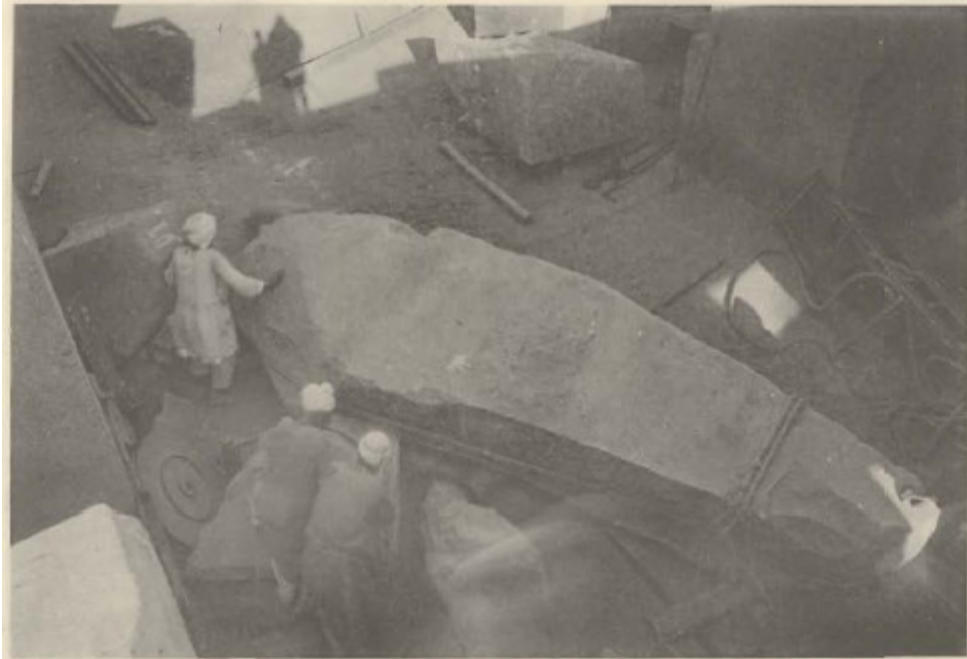
1. Removal of Coping-stone from Central Hall
