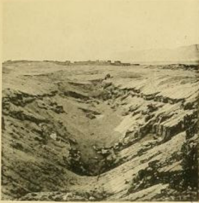
1. VIEW LOOKING SOUTH, SHOWING DIRECTION OF TRENCH.
