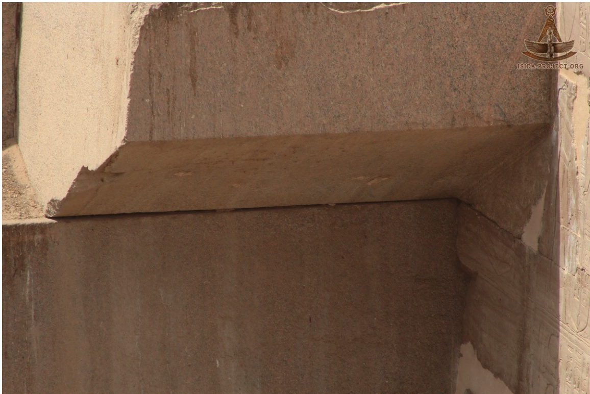
A closer view of the intact roofing beam
