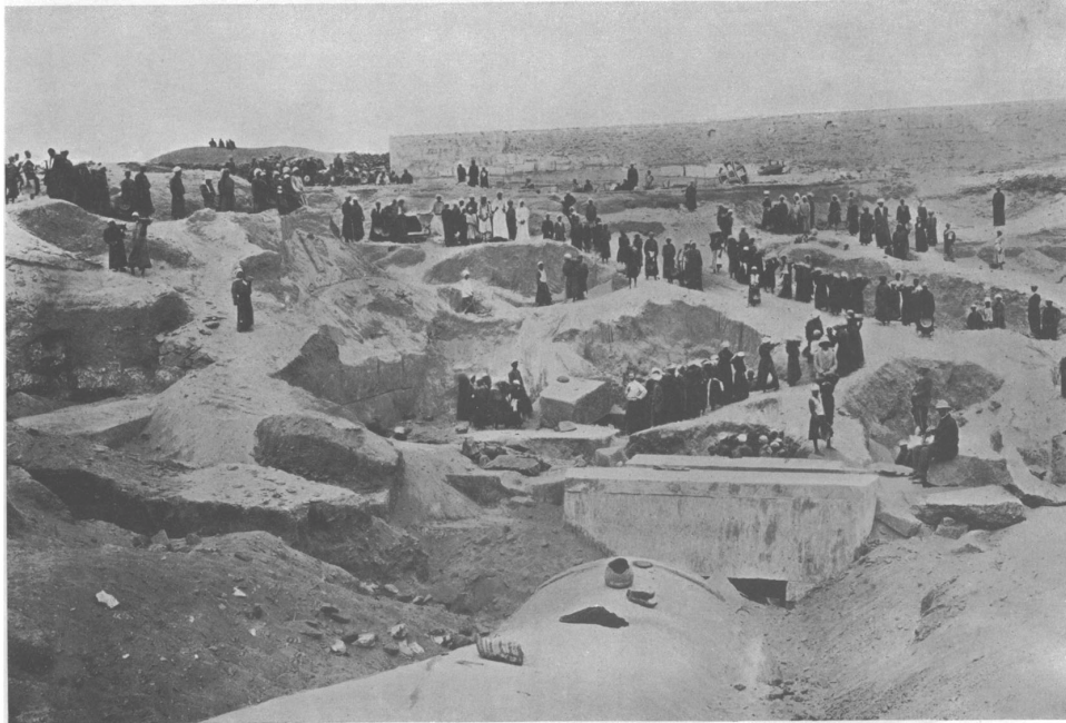
The Beginning of the Work: January 1914.
