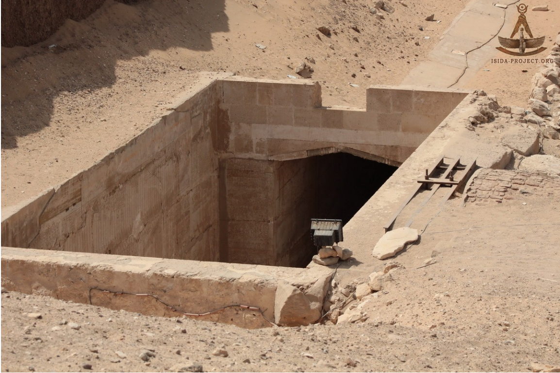
Modern view of entrance corridor entering into Great Hall, the modern arch that protects the sloping passage is visible on right
