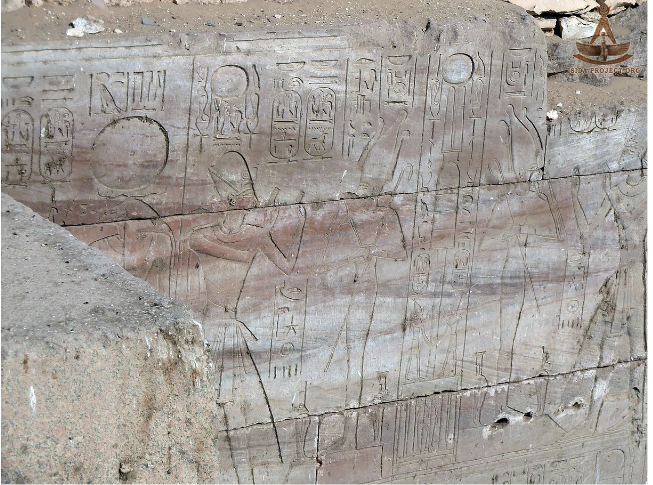
A close-up view of the decoration on top of the east wall
