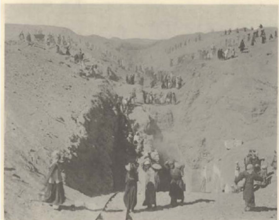
2. The clearing of the entrance passage with boys and gravity-railway, looking North
