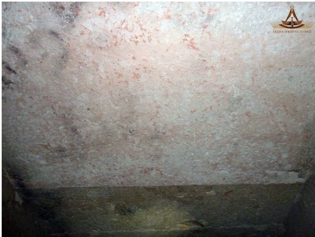
Construction lines can be seen on some of the ceiling blocks, along with red marks highlighting the smoothing process
