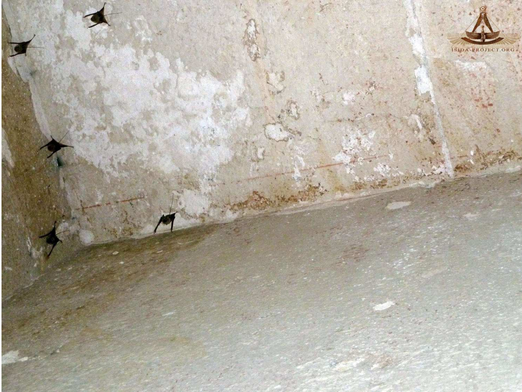
Construction lines can be seen on some of the ceiling blocks, along with red marks highlighting the smoothing process
