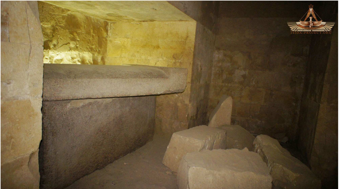
This view taken from the southern recess of the high hall shows its corresponding northern recess and sarcophagus recess. The ceiling height of the hall is an extra 5 cubits higher than the 4.5 cubit ceiling height for the rest of the chamber, giving the hall height as 9.5 cubits.
