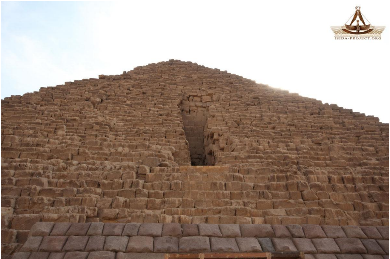
Image courtesy of Isida Project
