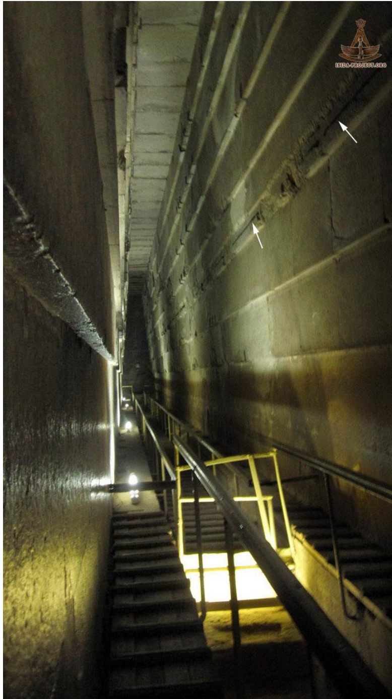
Image courtesy of Isida Project
