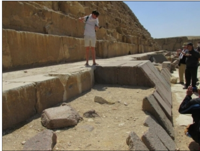
Granite casing stone of the Second Pyramid
