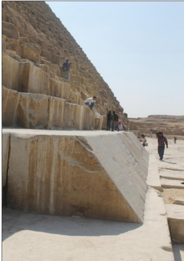
Remaining casing stone locking into the Great Pyramid
