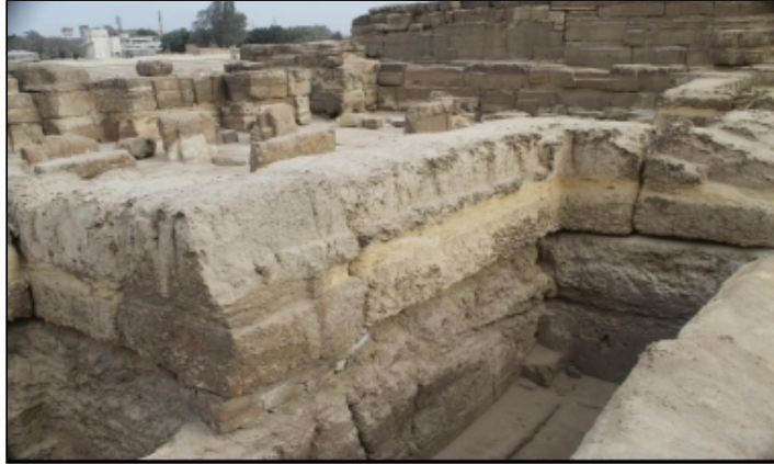
The Sphinx Temple blocks, put into place as cut from the enclosure
