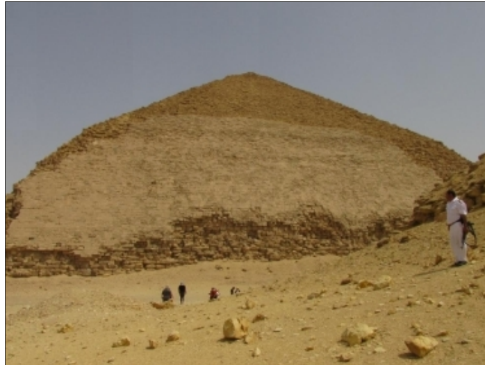
More casing stones missing from the upper half of the Bent Pyramid
