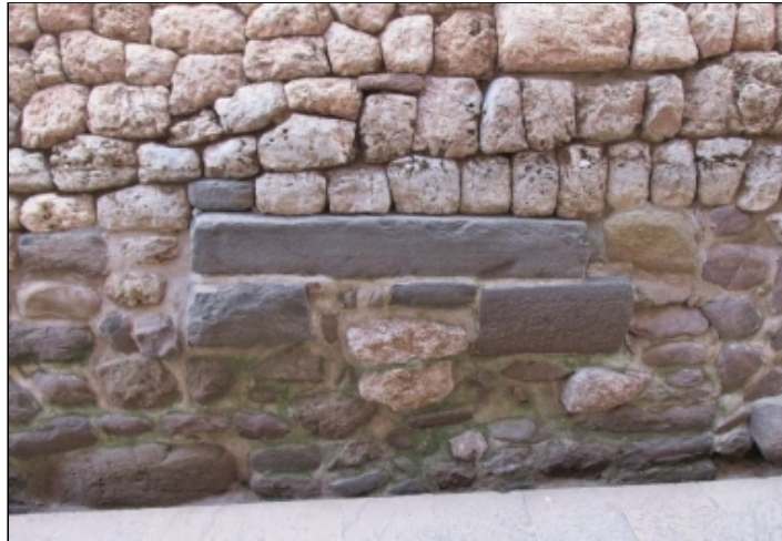
Inca wall with inserted megalithic basalt recycled stones
