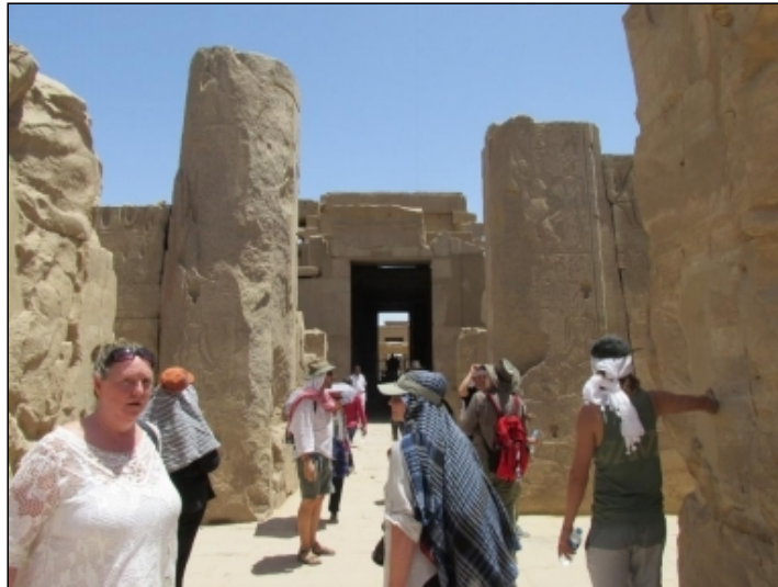
Damaged vertical stones on the left and right of the east/west path
