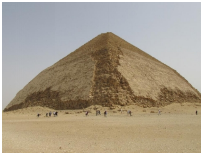
All four corners show extreme damage to the casing stones
