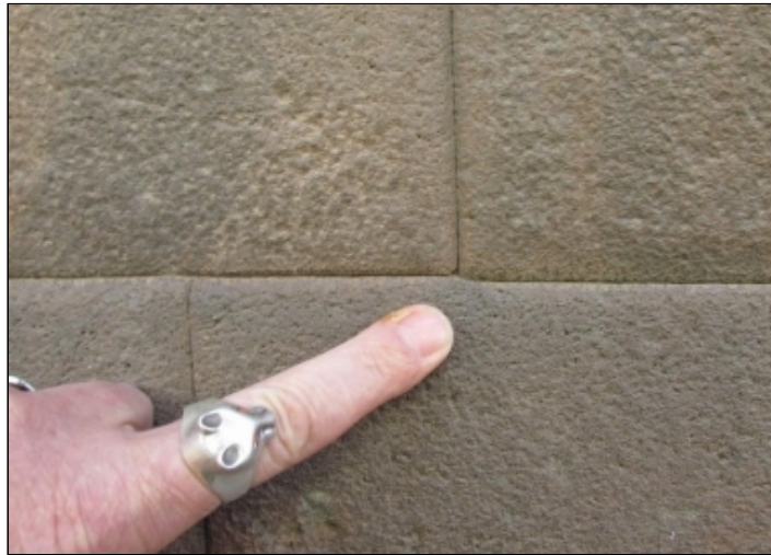
Astonishing accuracy of the Coricancha - the stone is basalt
