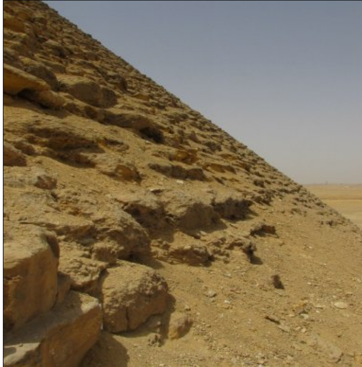
Appearance of extreme erosion on the Red Pyramid
