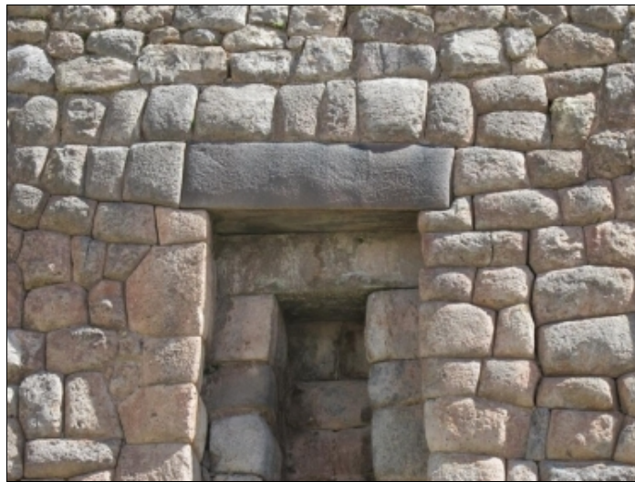
Manco Capac wall section with basalt lintel
