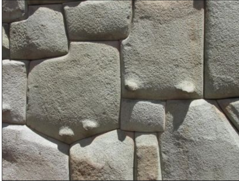
Inca Roca wall with amazing tight joinery
