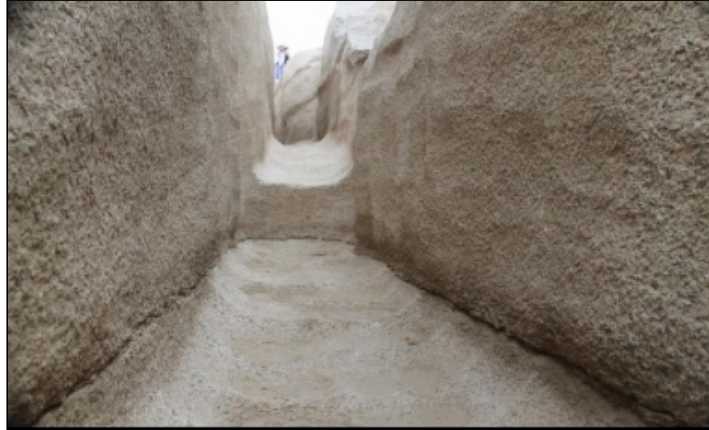
Crack in the bedrock in the right channel of the great obelisk
