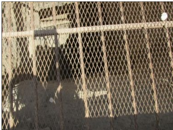
Looking down into one of the deep shafts
