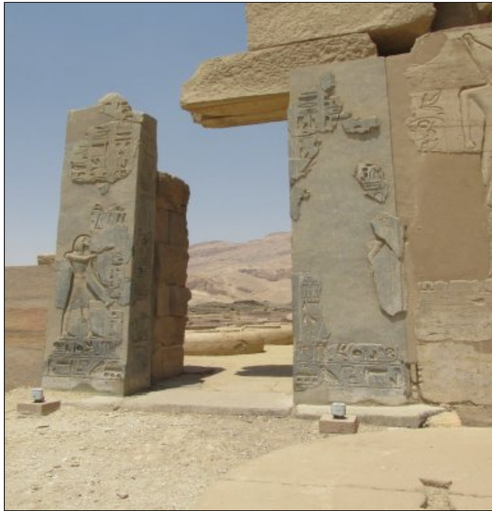
Badly disintegrated left gate that has been reconstructed
