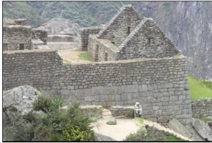
Machu Pic'chu: Inca repair work on top of older megalithic walls
