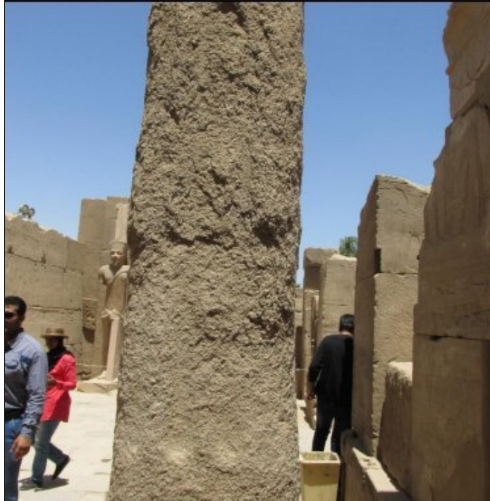
Extreme erosion on a vertical stone near the entrance to the Holy of Holies
