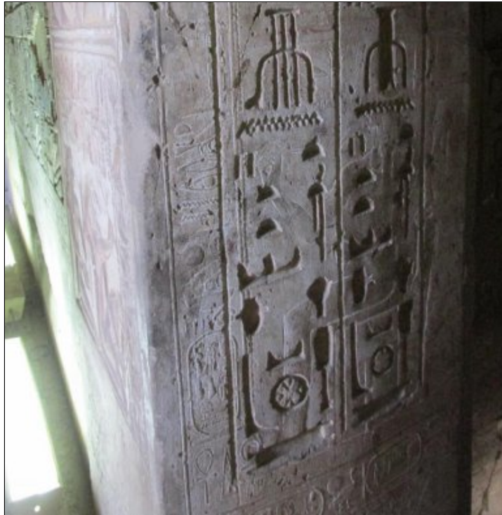
A wall section showing obvious evidence of recurring
