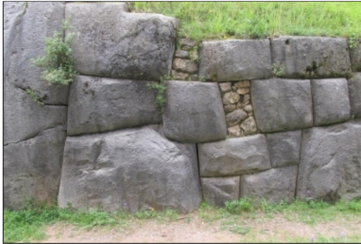
Megalithic work and smaller Inca repairs at Sachsayhuaman
