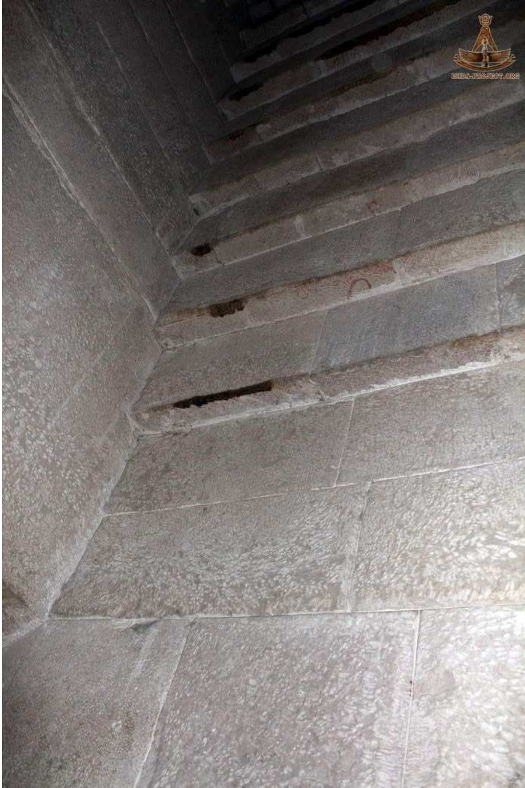
Looking up east wall, some mason graffiti can be seen on bottom face of corbels
