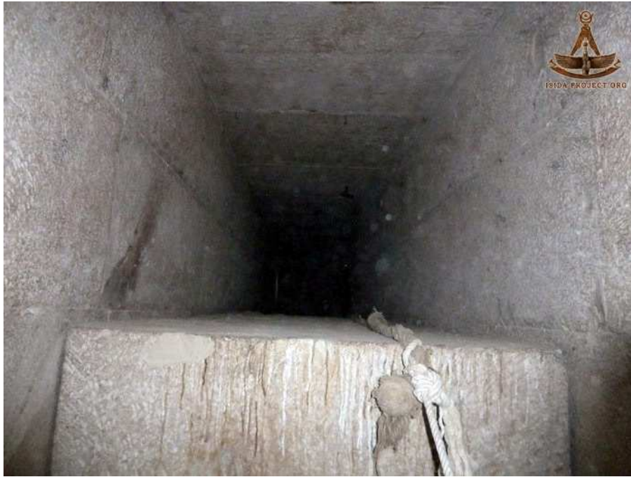
Top of plug block, the wall course joint gives a rough idea of height clearance afforded to the block on its journey down the corridor.
