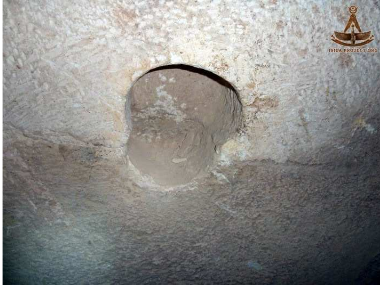
One of the holes in the corridor wall
