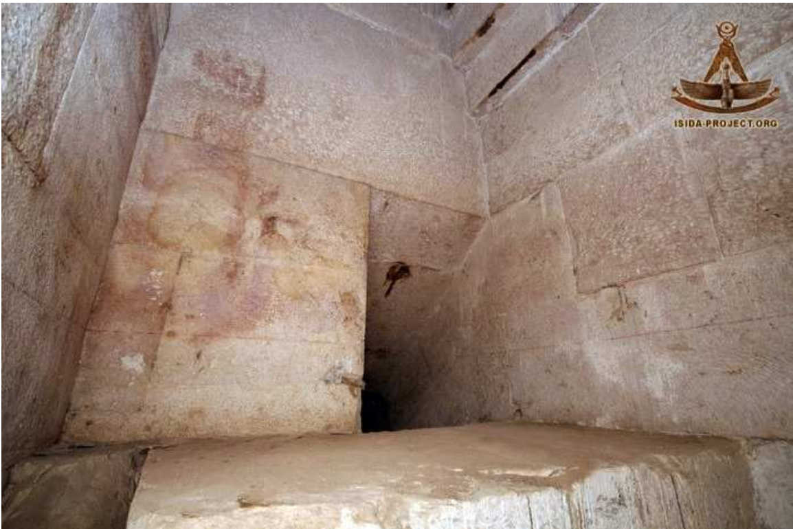
The large floor stone 1.18m thick can be seen in the foreground, also note the red level line running 1 cubit above this stone
