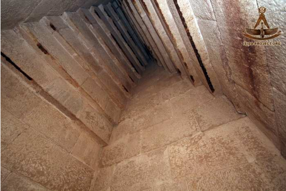
Looking up south wall
