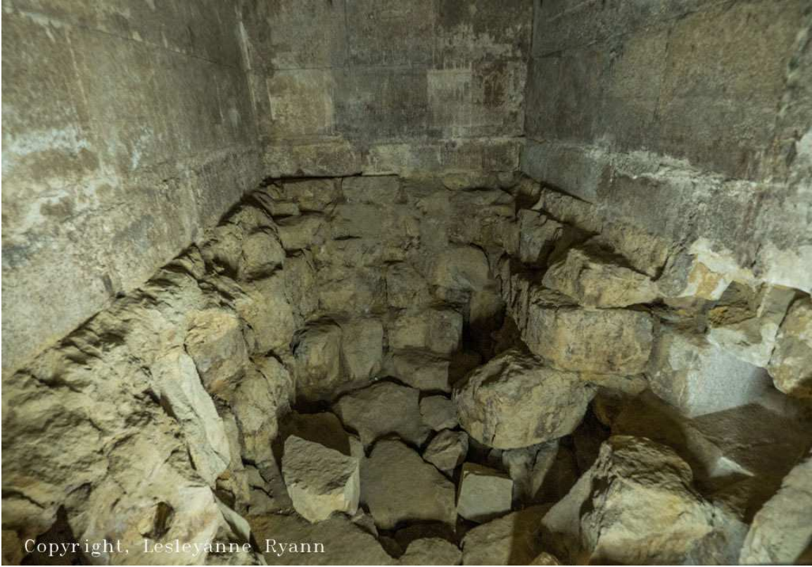
Excavation, showing breach in north wall
