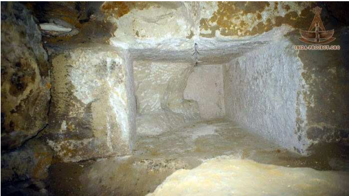
View inside north wall breach
