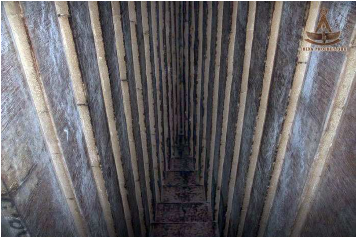
A view of lower chambers corbels
